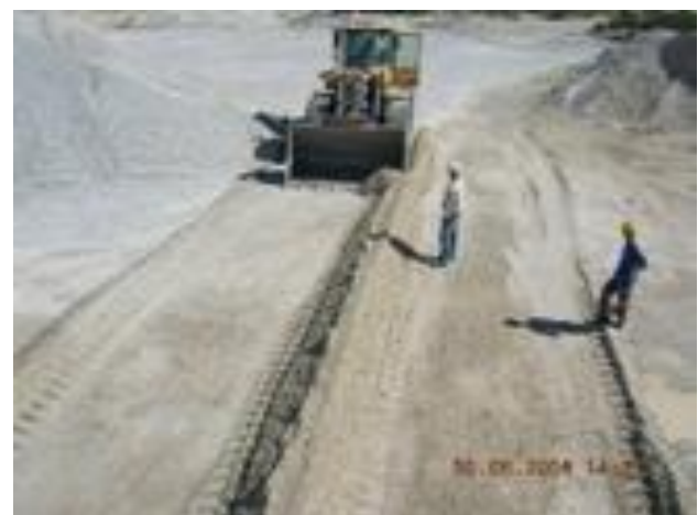
Front end loader levelling second (adjacent) bucket load
