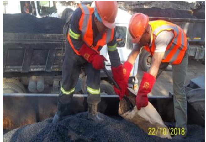
Figure A7: Asphalt Sample being Placed in a Sample Bag
