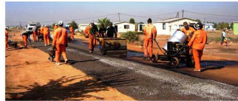
SURFACING OF A GRAVEL ROAD USING LABOUR BASED TECHNIQUES
